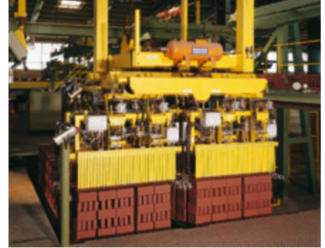
Stainless steel flexible tubes and bellows units at the kiln in the brickworks
