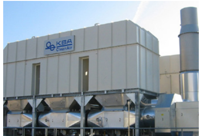
Incineration installation for thermal regenerative flue air purification
